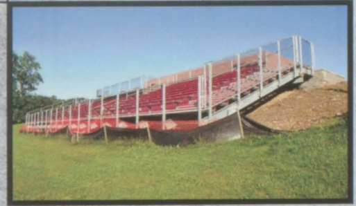
New bleachers were installed at Blackhawk Stadium.
